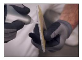
In case of a double pipe, drill a hole with the same diameter as the pipes at all the marked points, adding 15 mm. If the pipes are on the long side of the board, make a 45 degree cut from each hole to the side of the board.
