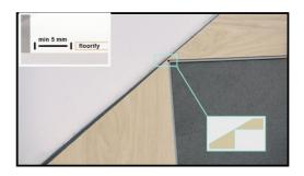
6. Place the various triangles with their corners against each other. Take the expansion joint into account and keep a minimum distance of 5 mm from the wall.
